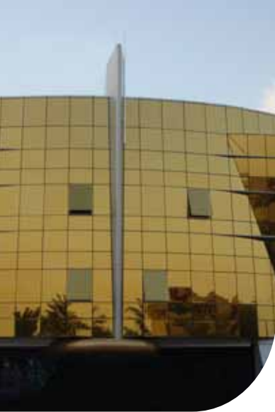
MKT Commercial Building Doha-Qatar Pilkington Eclipse™ Gold
